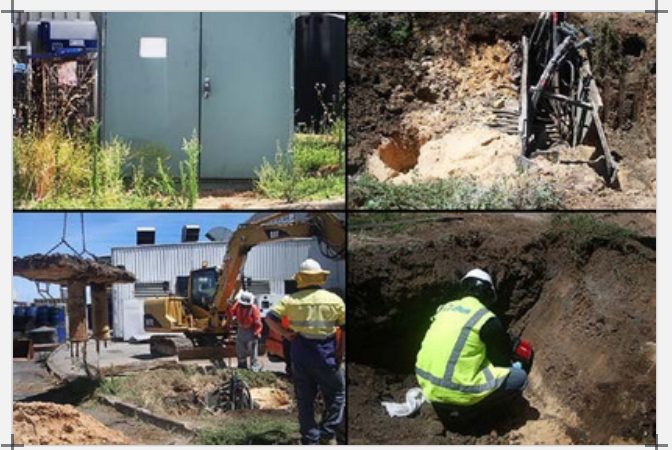
Excavation of the transformer footings, with RemScan measurements directing the extent of the dig.
