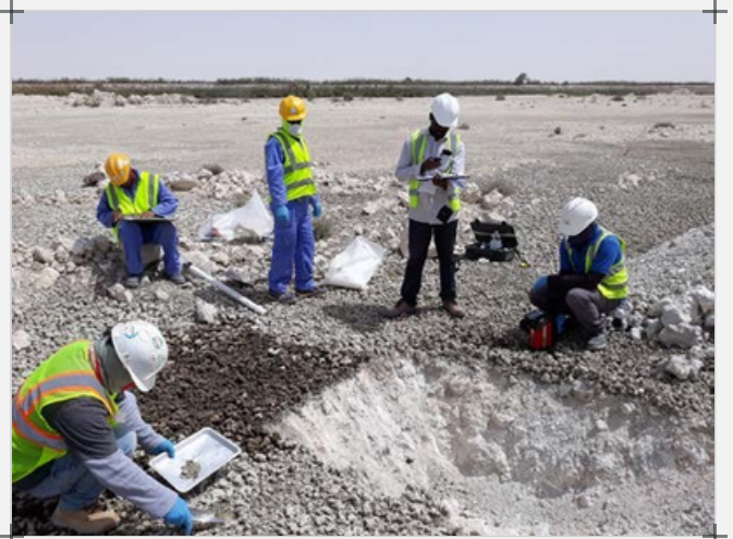
SUEZ monitoring TPH during excavation of the polluted sediments.
