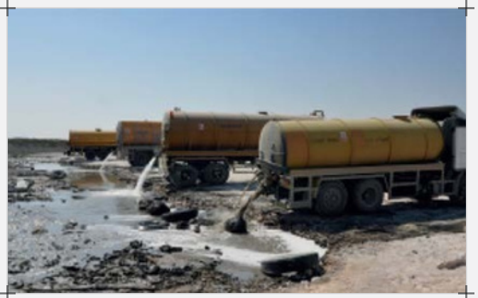
Tankers discharging wastewater into the lagoons, prior to remediation.
