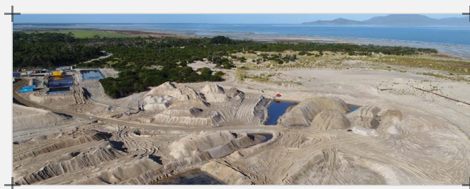
The protected foreshore site under remediation. Photo courtesy of Cardno.
